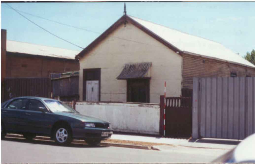
Figure 1: 15 Quebec Street, Port Adelaide. The site of the first excavation (Photo: Susan Briggs)
